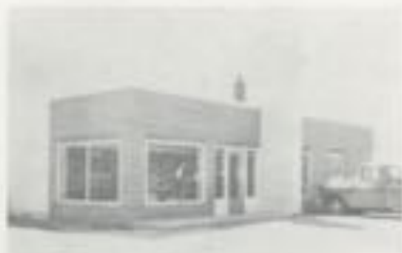
ARTHUR LUMBER AND COAL CO.
