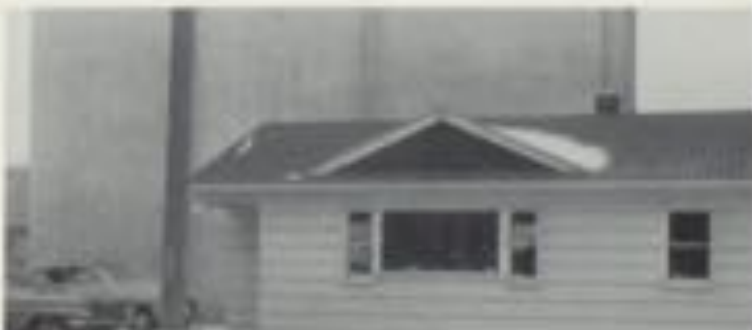
ARTHUR ELEVATOR COMPANY Arthur, Iowa
