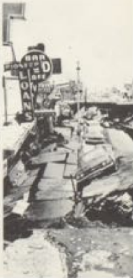
Alaskan Quake —A whole line of cars fell about 20 feet below street level on a main thoroughfare in Anchorage the day following the disastrous earthquake on March 27.
